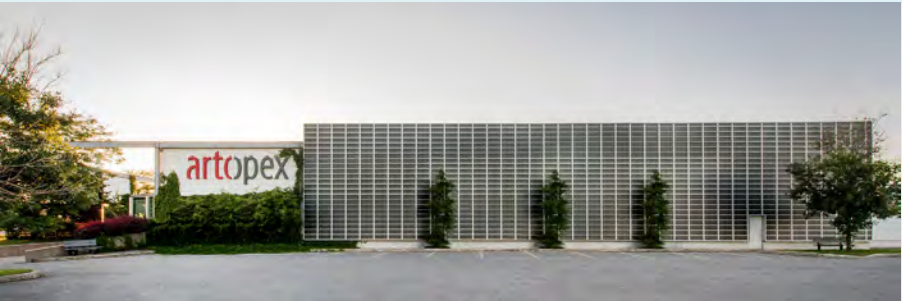
Solar wall on the facade of the metal furniture and components production unit Artopex Plus, Laval, Quebec
